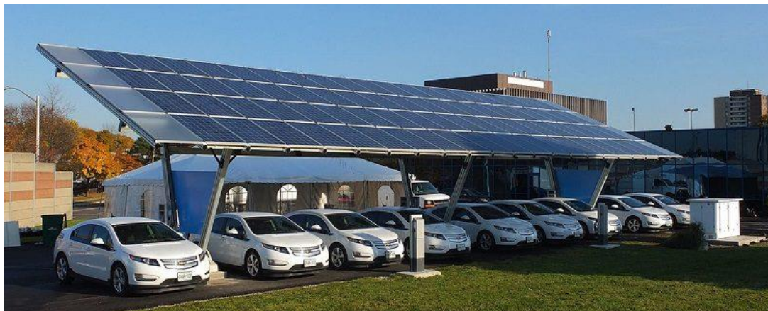
A solar charging station (Reference: Sinovoltaics )
